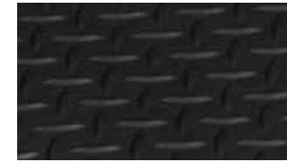
Deck top surface
